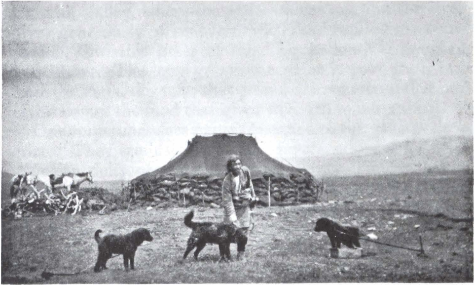
‘ The walls may be of sods with a roof of yak hair ’
